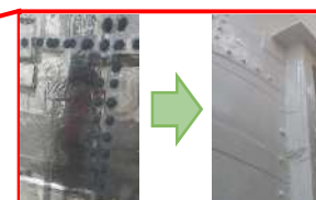
Covering by Titanium foil Top coating
