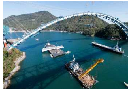
Engineering work in the port ( Misumi/Kumamoto )
