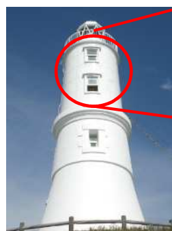
Covering by Titanium foil Top coating
