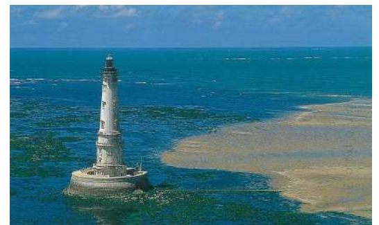
Cordouan Lighthouse (France)
