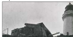
【Destroyed LH and the new LH (Yokosuka)】
