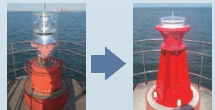
Reinforcing a light source against wave damage
